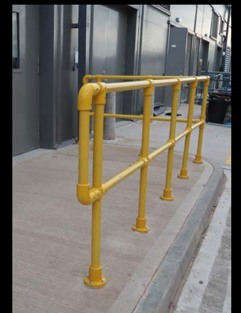
Handrailing: Ramp building access with key clamp handrailing.
