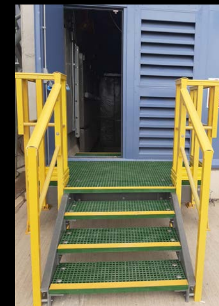
Stairs: Plant access up & over stairs to bund and building areas.
