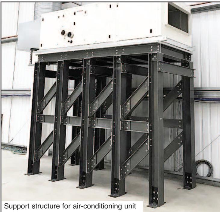
Support structure for air-conditioning unit
